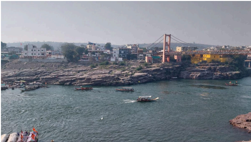
Hanging bridge from other side
